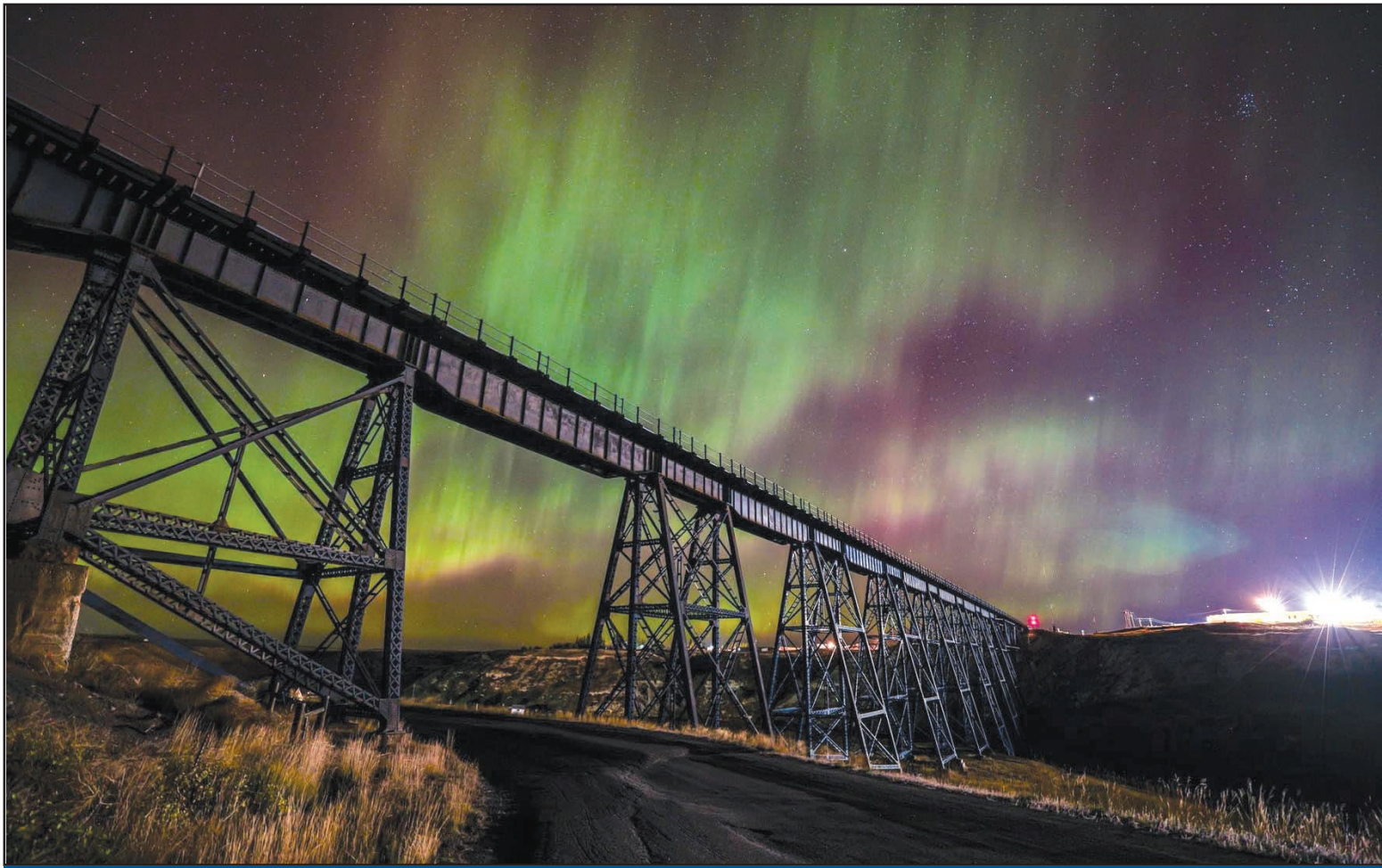
Jason Berg , a conductor for Amtrak out of Local 117 in Shelby, Mont., got this shot of the Cut Bank trestle on the hi-line near Cut Bank. The 124-year-old bridge was completed in 1900, stands 160 feet high and spans 1,200 feet.
