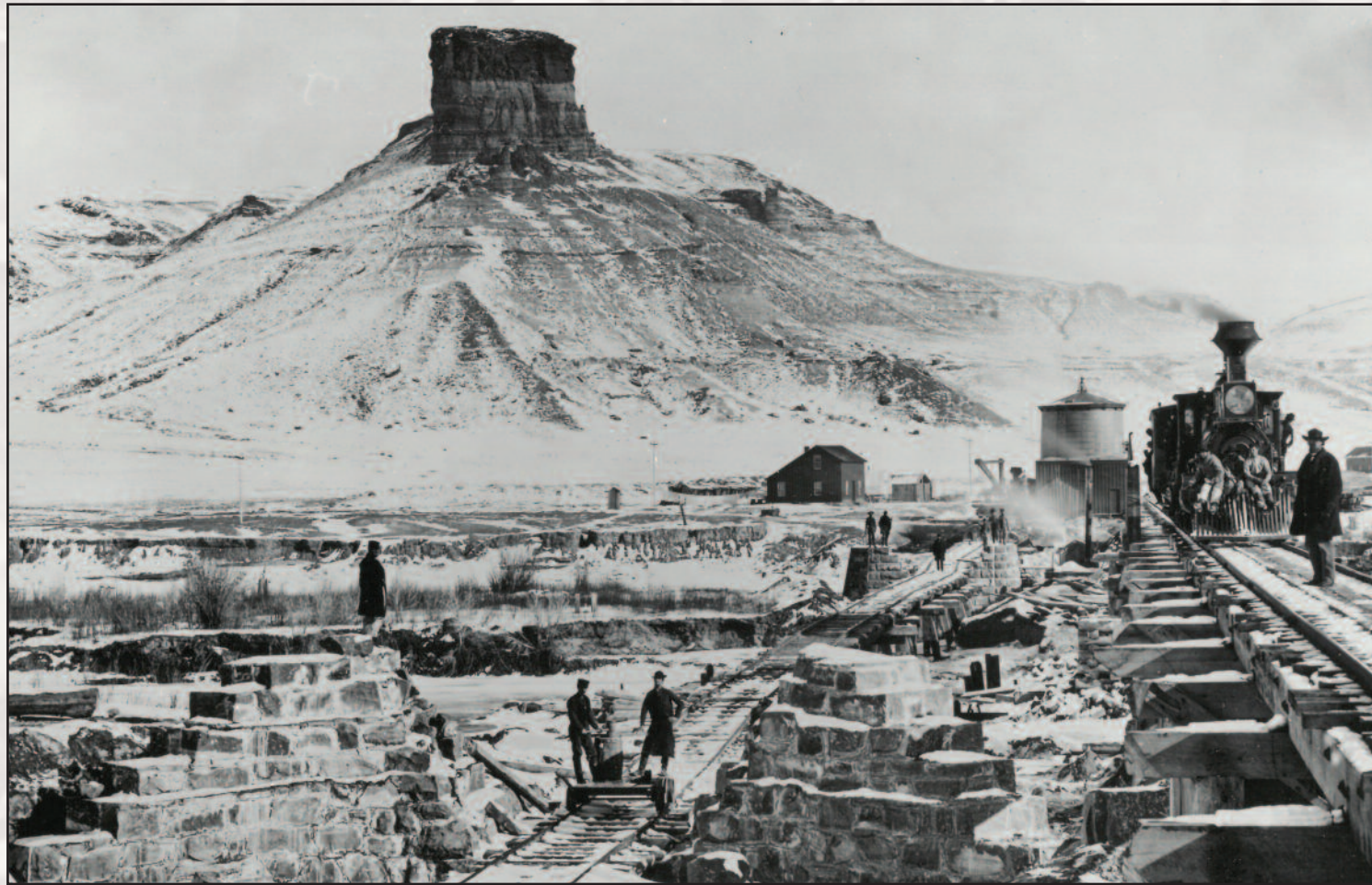
This bridge-building scene at Green River, Wyo., taken in 1868, is one of photographer Andrew J. Russell's grandest photographs. Temporary and permanent bridge structures over the Green River are shown in the foreground while the magnificent Citadel Rock rises high in the background. A work train is on the temporary wooden bridge at the right unloading stone for use on the permanent bridge supports rising on the left. The hazardous work was made even more dangerous by snow and ice as the Union Pacific crews worked right through the winter in their rush to beat the Central Pacific to Salt Lake City. The advance rail layers had moved westward toward the Wasatch Mountains and this photo shows the follow-up crews working on installing more permanent structures.
